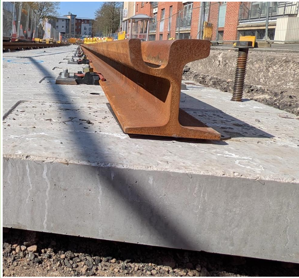
Step #4 Rail delivery, cutting and setting out
