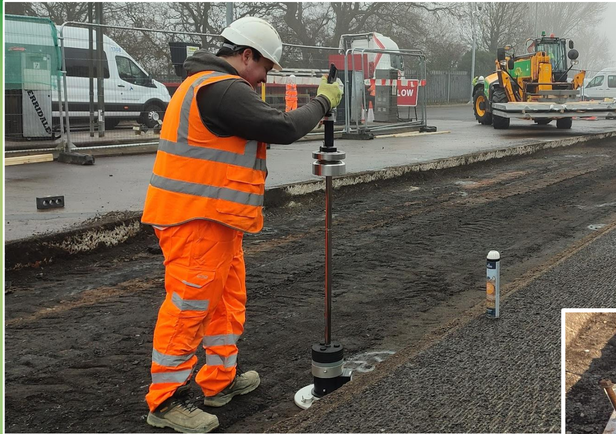
Step #2 Surface bearing capacity quality control, rebuilding of top section of access chambers and preparation of rail water drain connections
