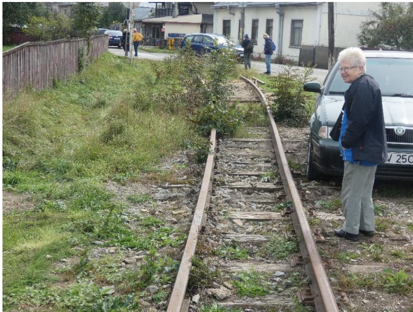
Fig.17. The transition from 760mm gauge to standard gauge at Vatra Moldovița. The track in the foreground is 760mm, but through the bushes, there is a gradual widening to link the narrow-gauge rails to the track on the now-closed standard-gauge branch from the mainline network to Moldovița. (Photograph: David Murray-Smith).
