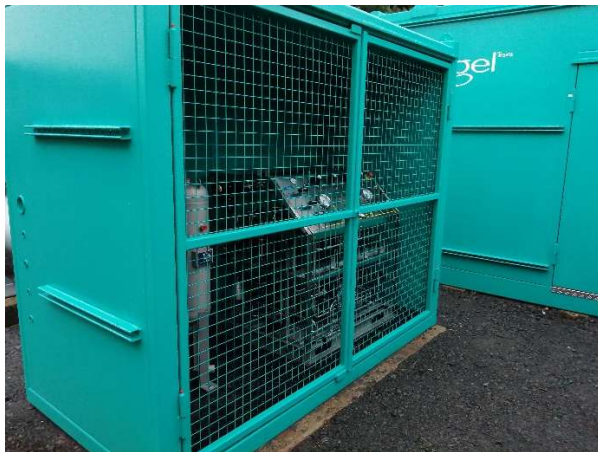
Figure 9. Electrolyser and refuelling equipment at Bo'ness station.
