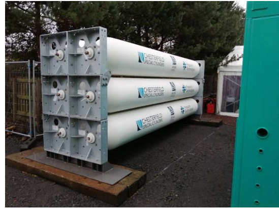
Figure 8. Hydrogen cylinders forming part of the facilities for refuelling at Bo'ness station.
