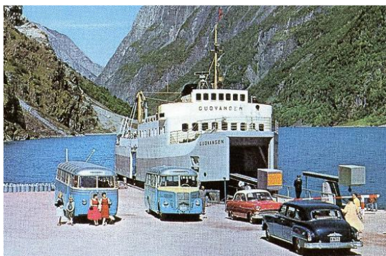
Norway 1954 – Gudvangen 30 cars, 10 crew Drive-through at 'lock-on' linkspans
