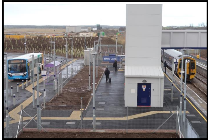
Inverness Airport station and bus bay. The total cost for the entire project and wider associated works was £42 million. Photo: Neil Wallace
